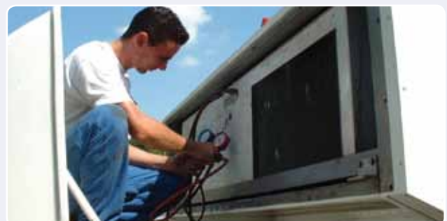
Inspection of refrigerant circuit
