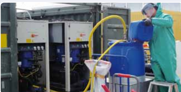
Cleaning of chilled water circuit
