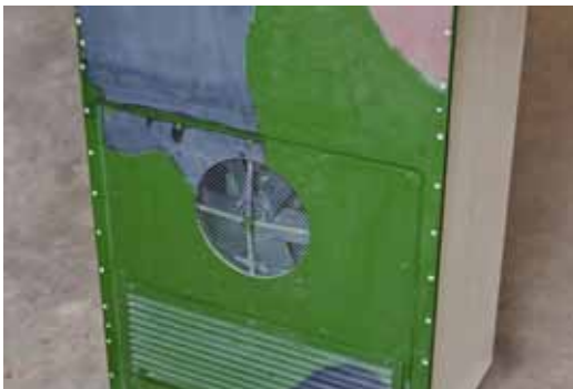
Air-conditioning unit for shelter
